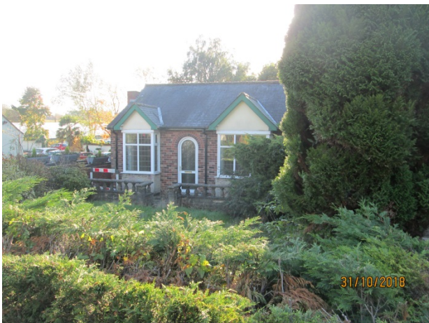
Front of existing dwelling.
